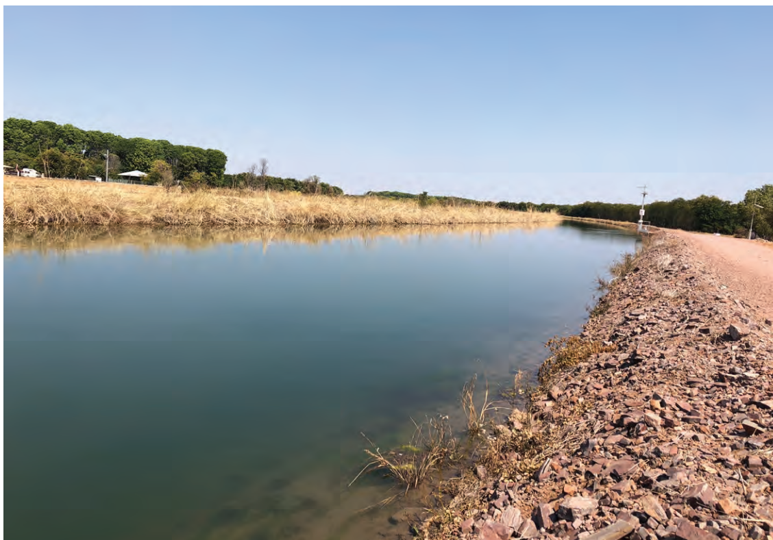
Figure 4. An agricultural water channel (unlined).
