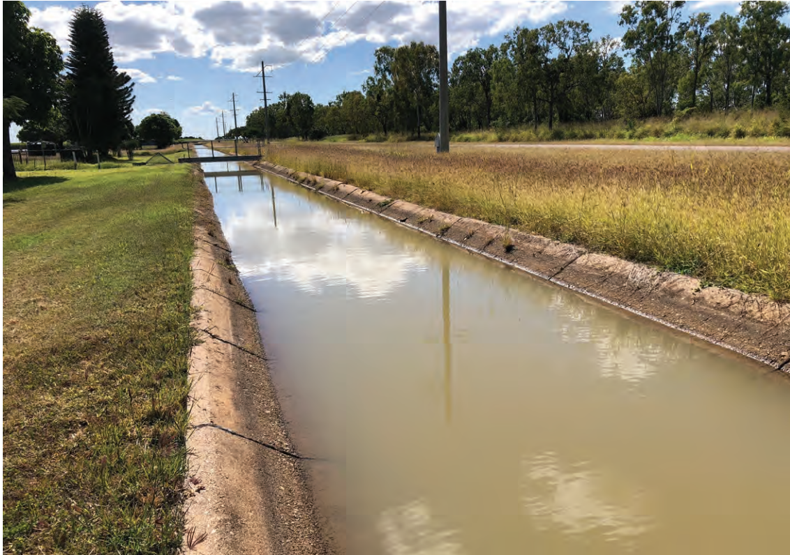
Figure 5. A concrete-lined agricultural water channel.
