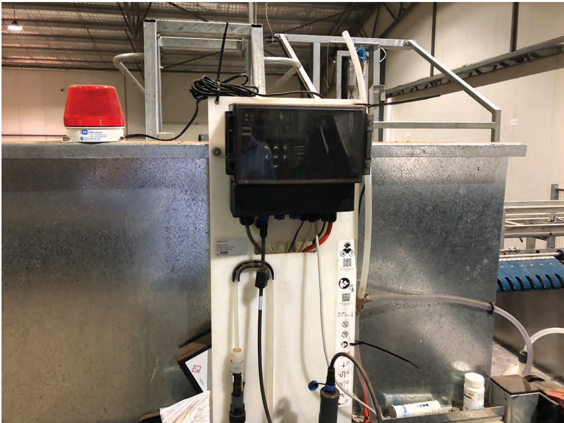
Figure 23. An automated monitoring and alarm system to manage sanitiser levels in a dump tank.
