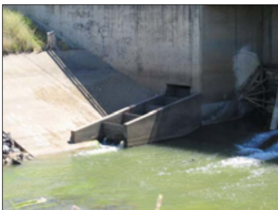
Figure 2. A) and B): submerged-orifice fishway, Tareelaroi Regulator.
