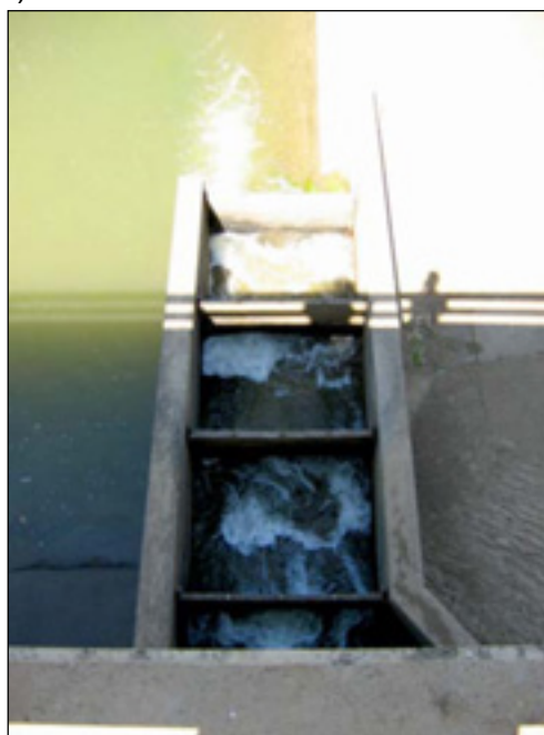
Figure 2. A) and B): submerged-orifice fishway, Tareelaroi Regulator.
