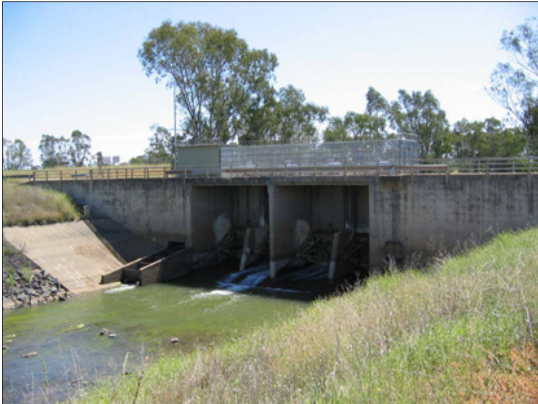
Figure 1. Tareelaroi Regulator, Mehi River view of weir from left bank (29.751ML/day).
