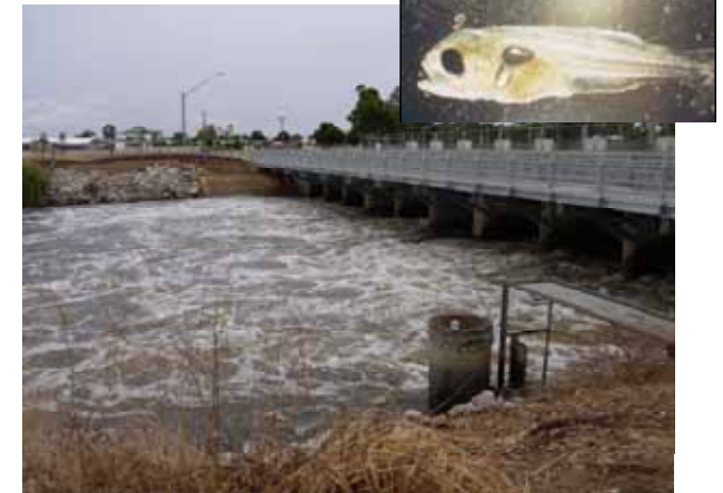
Downstream of the Mulwala Irrigation Canal inlet regulator. Native fish larvae (pictured) are mostly killed when they go through this type of structure. Photo: Jodi Frawley. Larva photo: Lee Baumgartner.
