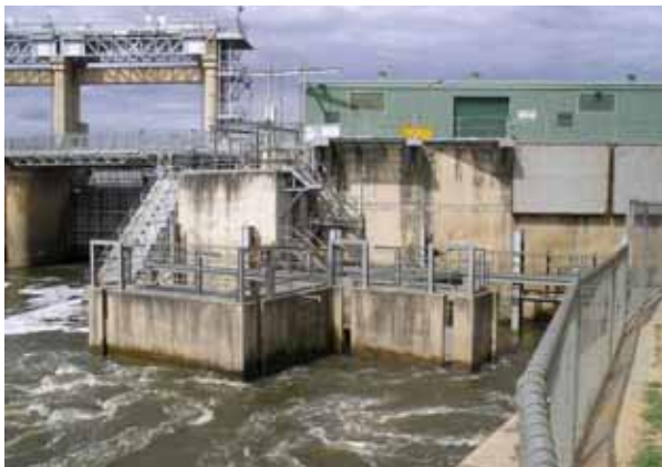
Encased in all this concrete is a 'vertical slot fishway' that allows larger migratory fish like Murray cod, trout cod, golden perch and silver perch to migrate past Yarrawonga Weir. Photo: Scott Nichols.
