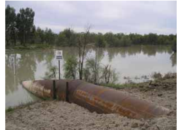
Irrigation offtake Tandou Creek. Photo: Scott Nichols.
