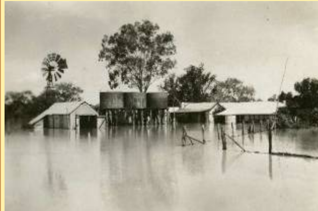
1942 flood - The Flat and Tanks. Photo source: Colin Leigo.
