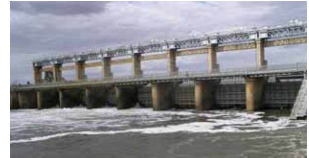
Yarrawonga weir, viewed from the downstream side, creates Lake Mulwala. Photo: Scott Nichols.
