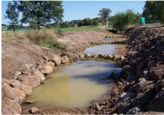
A 'chain of ponds' was created in the creek to slow water and aid sediment deposition.
