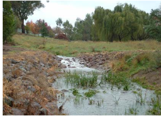
A rock chute was also installed to prevent bed erosion.
