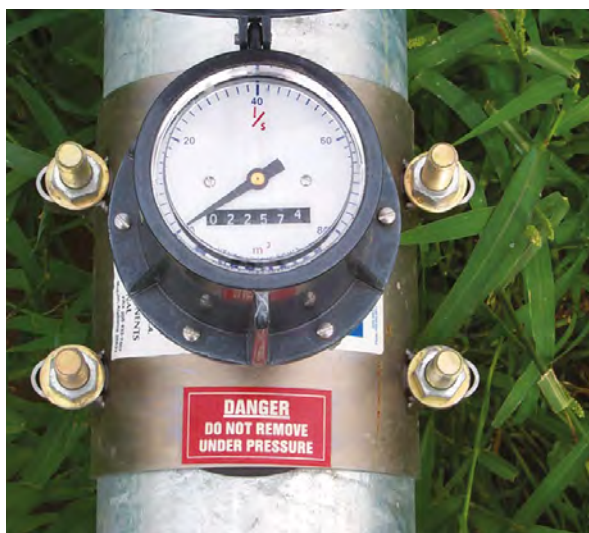
Figure 47. Flow meters provide an accurate record of water delivery to the orchard.
