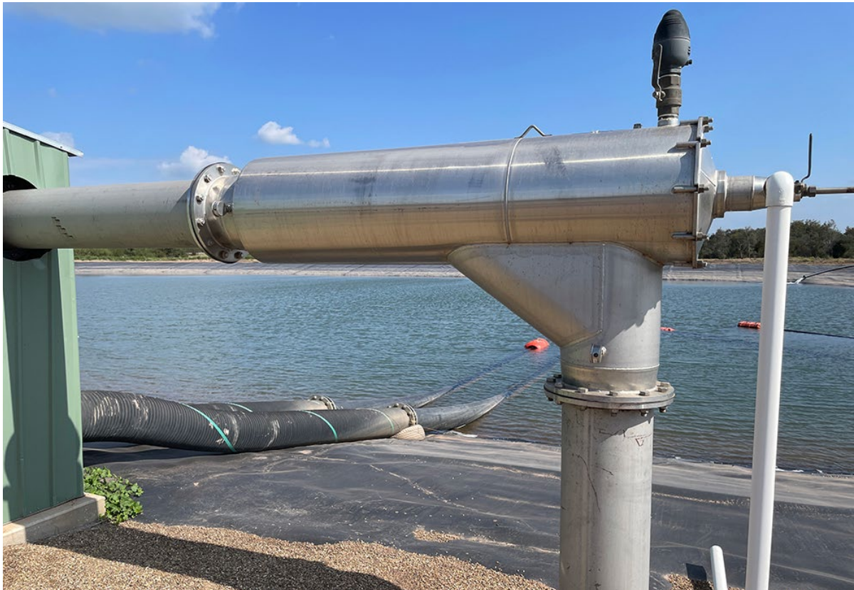
Figure 4. Using coarse filtration and frequent backflushing minimises the sediment and reduces the microbial population in irrigation water.
