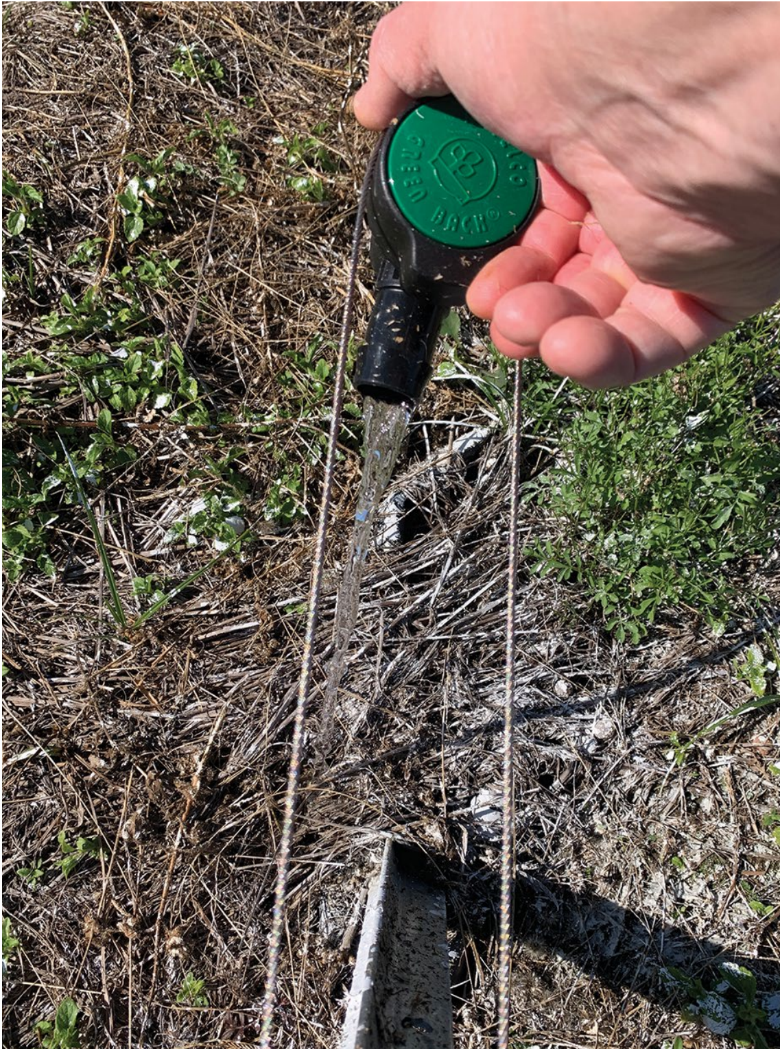
Figure 32. Flush the system (lines and filters) regularly to reduce blockages.
