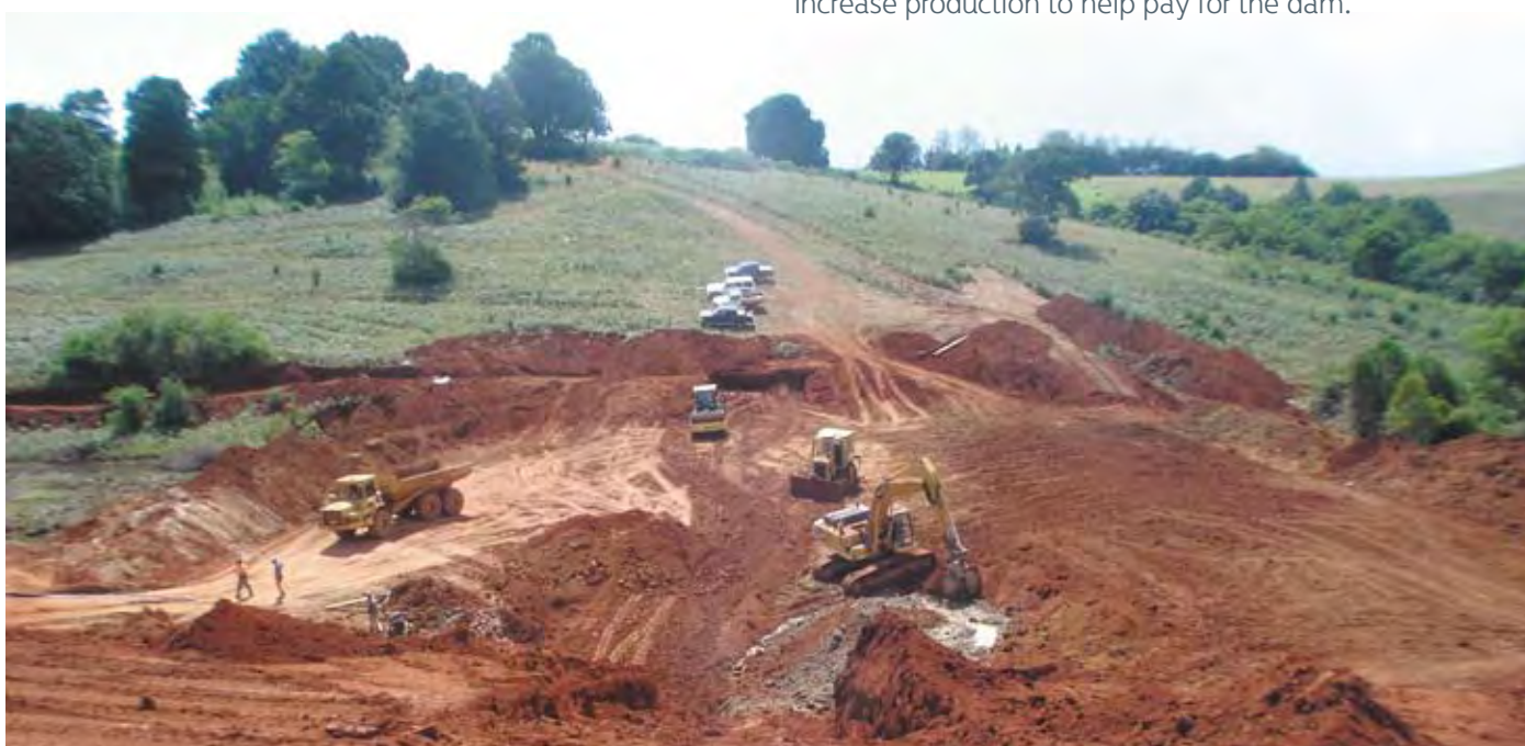
A new irrigation dam under construction. The design should be prepared by a qualified person and should be based on proper soil tests, especially for the dam embankment. Bypass capacity must be high enough to cope with extreme storms.
