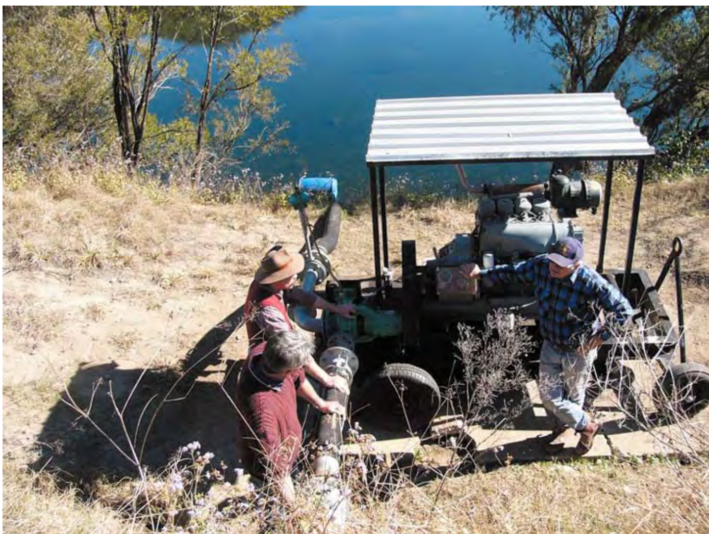
This portable pump unit, situated low on the Clarence River bank for maximum efficiency, provides water for a broad area cropping system and can be easily moved away from flood damage.
