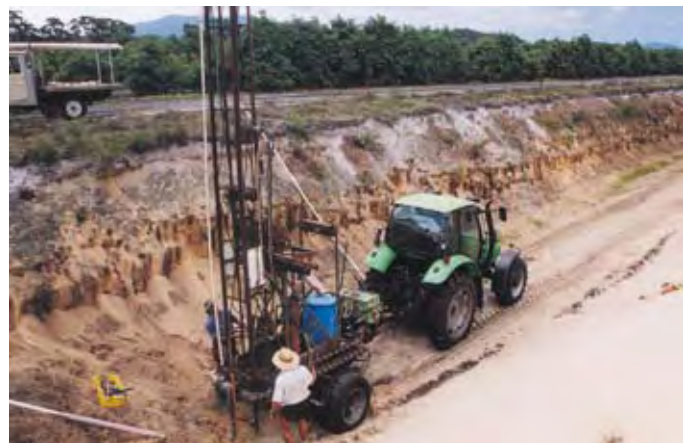
Drilling to establish a groundwater bore to irrigate avocados.
