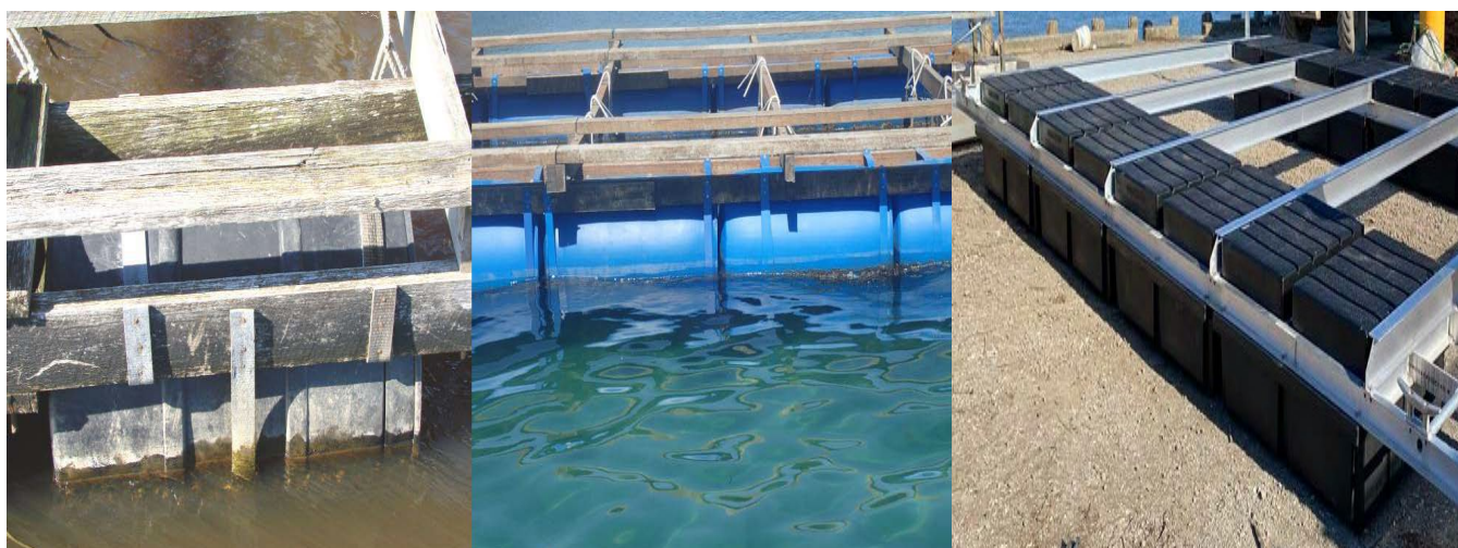
Figure 8. A 200 litre plastic drum secured to longitudinal raft timbers by two cushioning top shoulder straps and a drum girth strap (left). A 200-litre plastic drum secured to longitudinal raft timbers by two drum girth straps (centre). Eight 600 litre rota mould floatation devices bolted into the frame of an aluminium raft (right). Image source NSW DPIRD Aquaculture Management and Armstrong Oysters.
