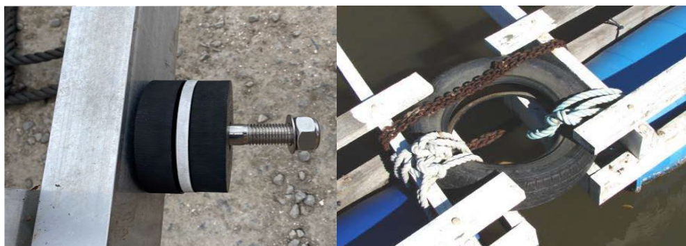
Figure 12. Shock absorber connected to aluminium raft join (left) and car tyre connected to longitudinal timbers either side of a timber raft (right). Image source NSW DPIRD Aquaculture Management and Armstrong Oysters.
