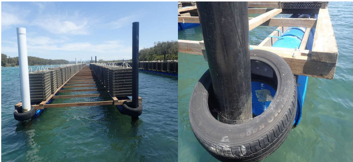
Figure 11. A post moored raft complex that has been approved by NSW DPIRD to incorporate white navigation marking on a raft directly adjacent to a navigation channel (left; see navigation marking requirements below). A car tyre sliding collar on a post mooring system suitable for use in shallow areas (right. Note: tyre double bolted internally through a reinforcing plate and reinforced raft module end plate). Image source NSW DPIRD Aquaculture Management.
