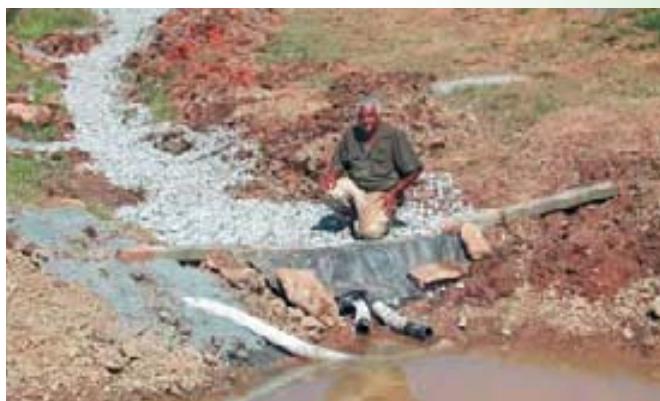
Figure 6: Sub soil drains were installed to flow into sedimentation pond
