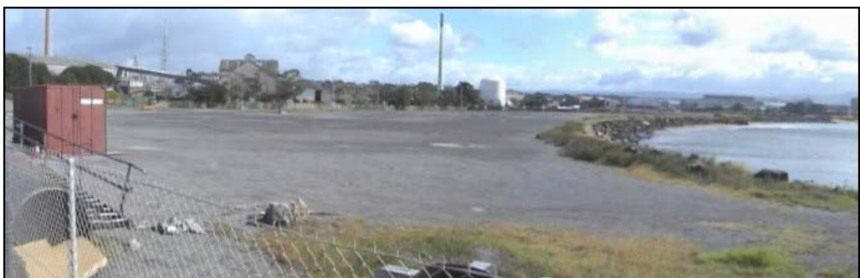
Cleared portion of 5A (Special Uses – Port) land adjacent to Jetty No. 3
