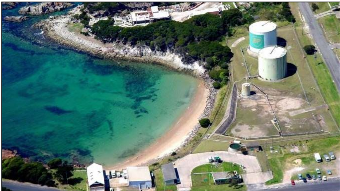
Aerial photograph of Yallumgo Cove and ex-BP site
