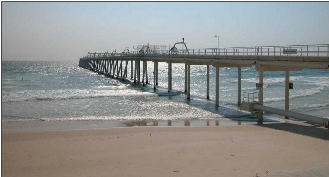
Re-watering Jetty, Tweed River Entrance Sand Bypassing Project
