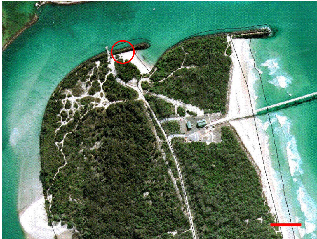
Aerial photograph of Fingal Peninsula, depicting sand bypass facilities and rewatering jetty (circled). Scale bar = 100m
