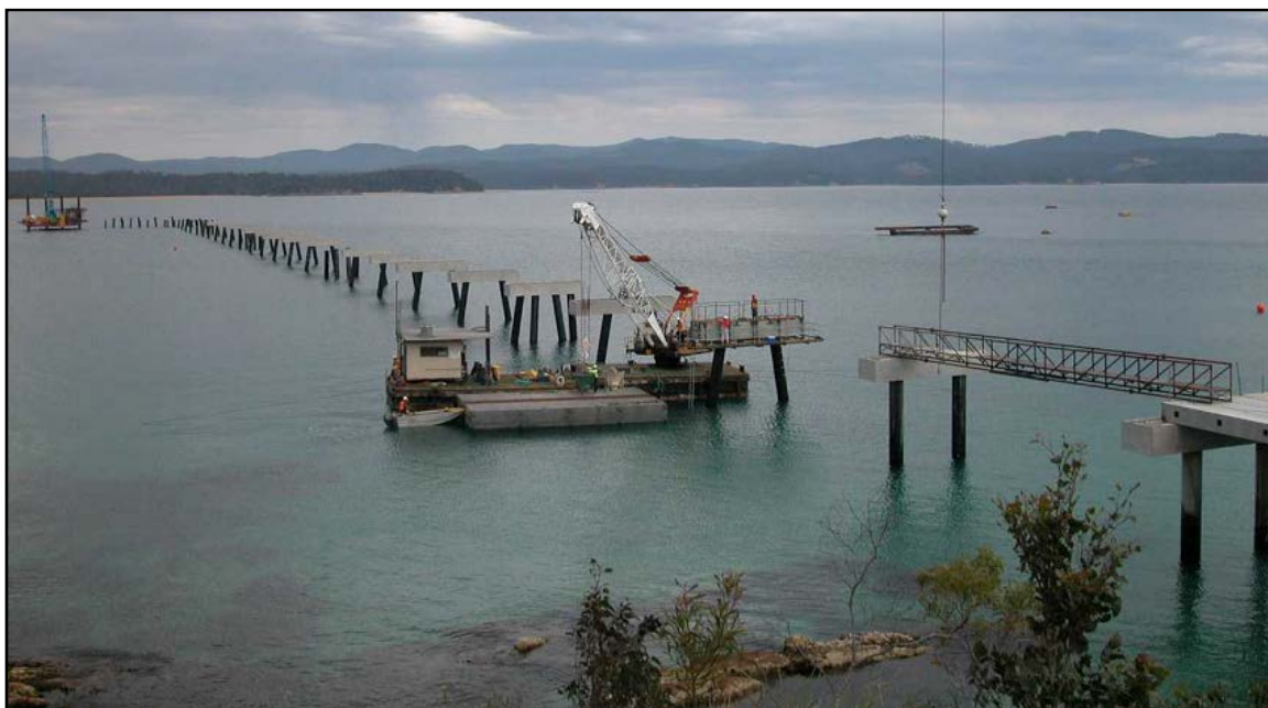
Twofold Bay Multipurpose Wharf (under construction)
