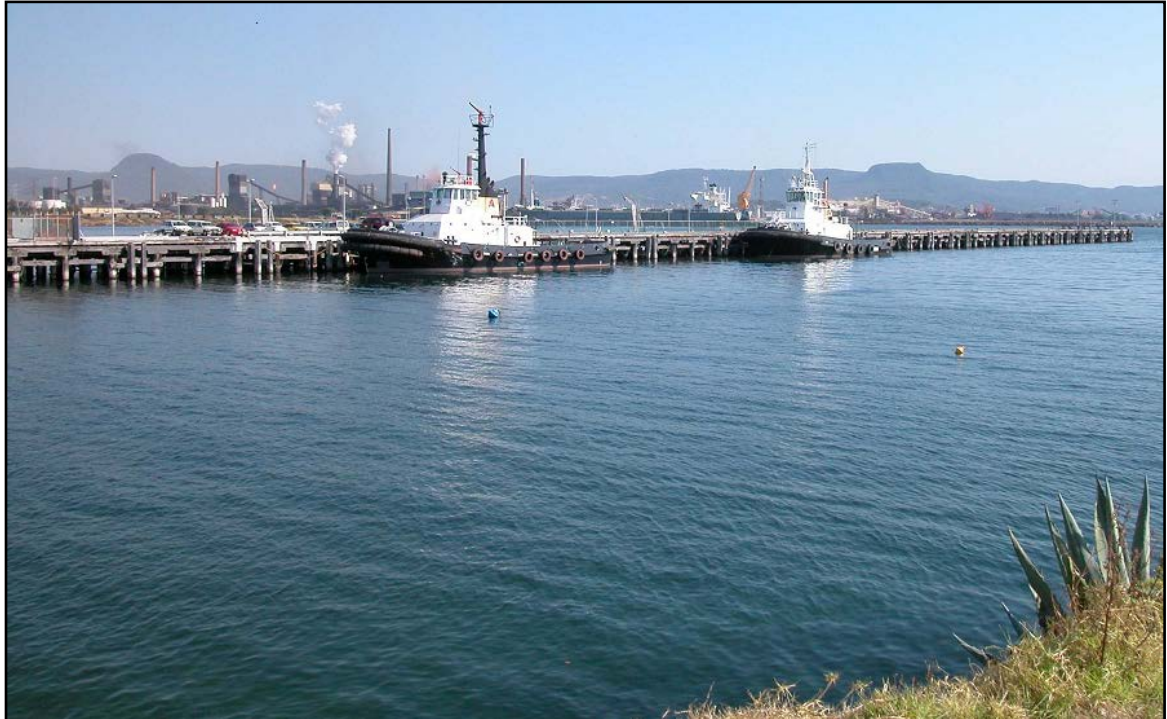
Jetty No.3, Outer Harbour Port Kembla, looking north-west towards the steelworks
