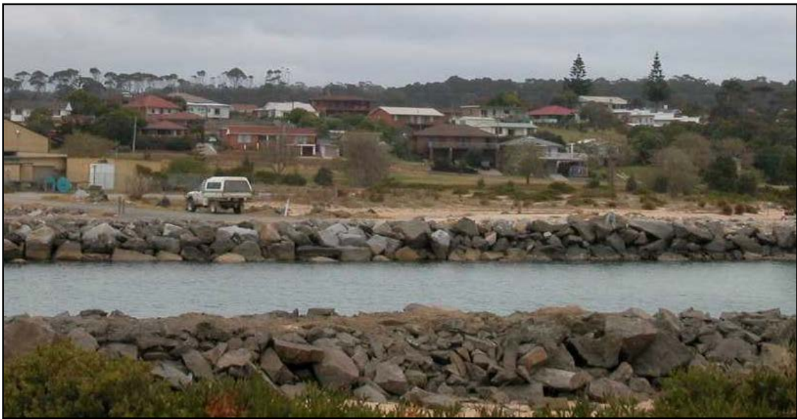
Bermagui Harbour, looking south to the shipwright sheds and adjacent vacant land
