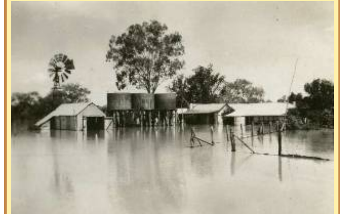
1942 flood - The Flat and Tanks. Photo source: Colin Leigo.
