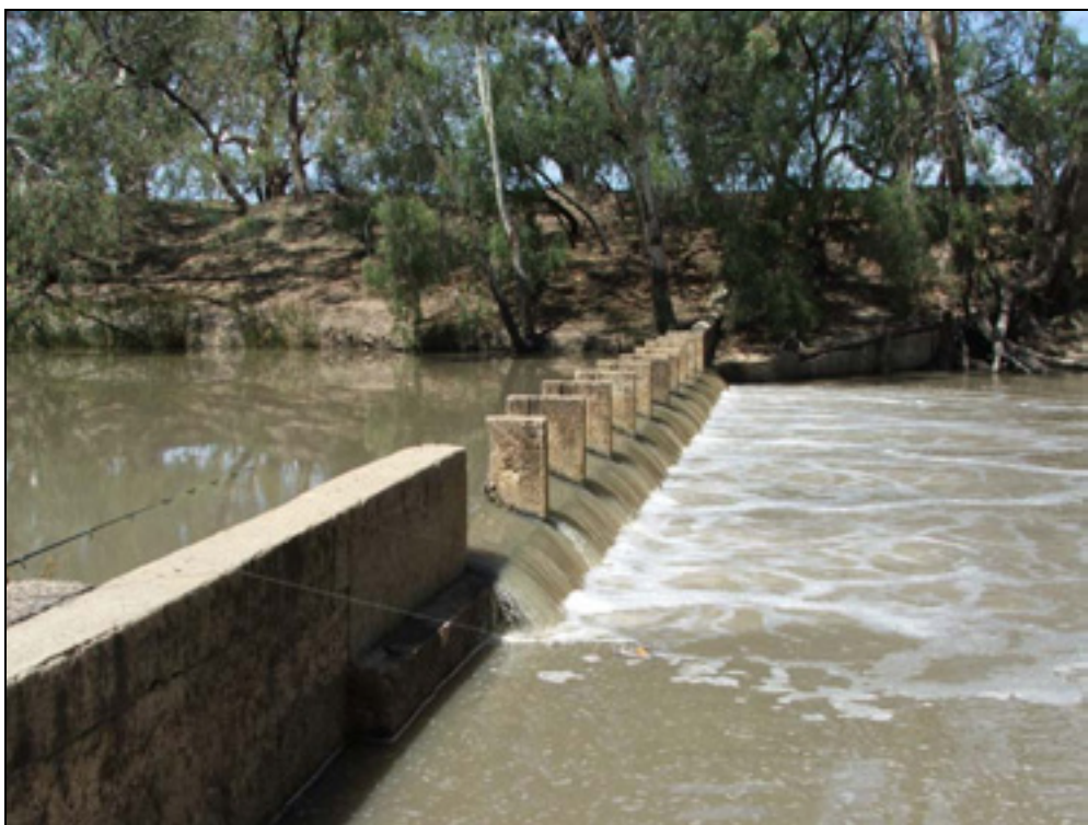
Figure 2. Wanganella Town Weir looking across the crest, Billabong Creek (04.03.2005, 142ML/day).
