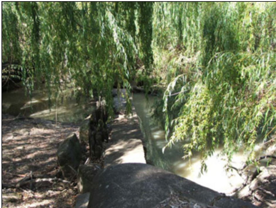
Figure 2. Road Paddock Dam (constructed 1915), Billabong Creek (07.03.2005, 98ML/day).
