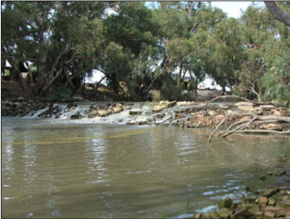
Figure 1. Jerilderie Town Weir (constructed 1894, last modified 1943), Billabong Creek (07.03.2005, 98ML/day).
