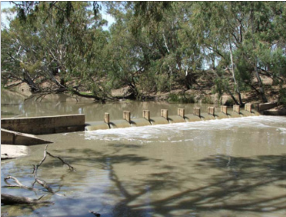
Figure 1. Wanganella Town Weir, Billabong Creek (04.03.2005, 142ML/day).
