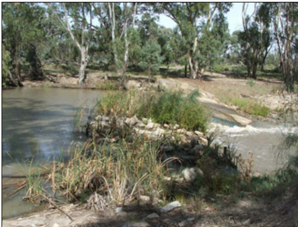
Figure 2. Accumulation of vegetation on Windouran Dam, Billabong Creek (04.03.2005, 142ML/day).
