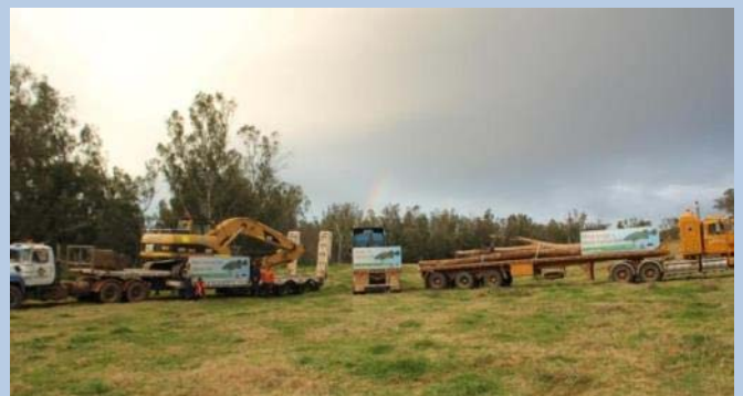
New fish habitat ready for installation.
