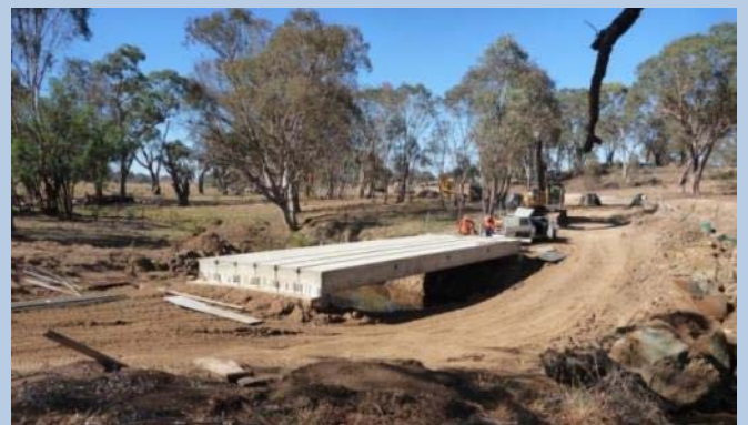
Construction works underway at Heads Road.
