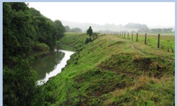
The next reach ripe for rehabilitation!
