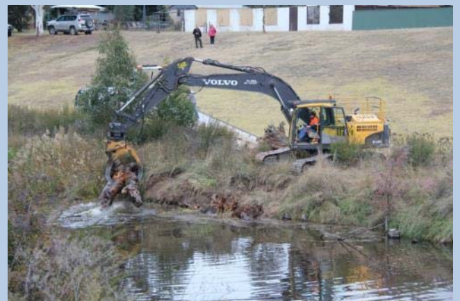
One of 20 snags being installed to provide habitat for native fish.
