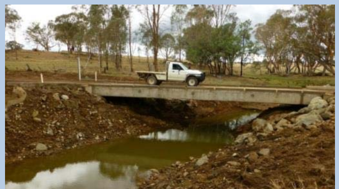
Improved access for fish and local residents.
