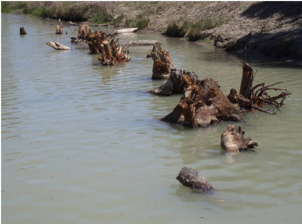
Figure 13. Large wood added to the river channel during re-snagging.
