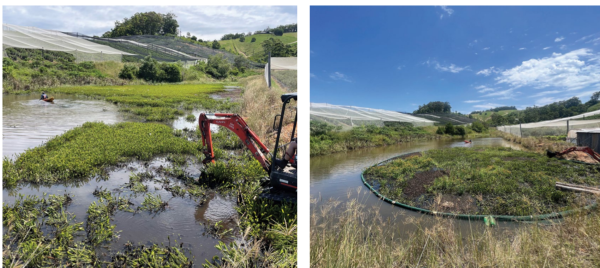
Figure 20. Mechanical removal of weed from a dam using an excavator and net.
