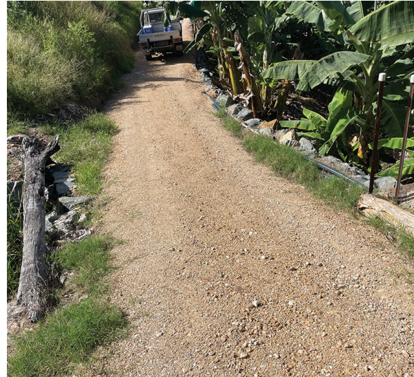
Figure 26. A compacted gravel driveway used to reduce erosion on the main track.
