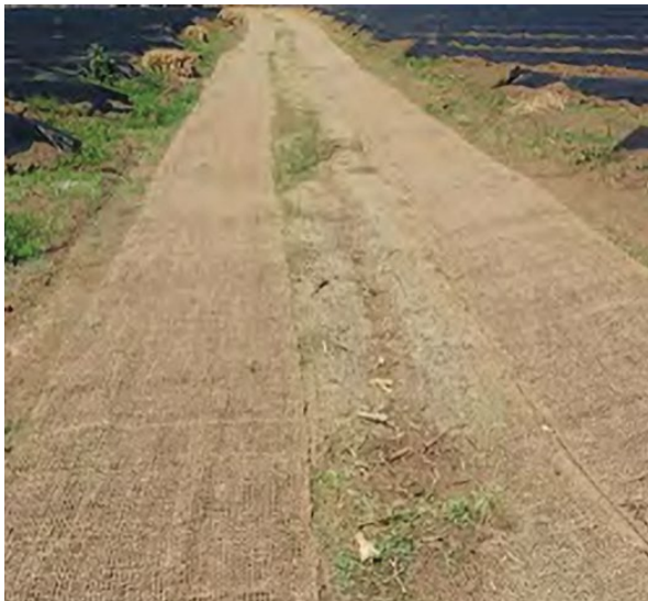
Figure 27. Jute mesh used to line a cross drain. Grass will grow through the mesh and break down afterwards. Photo: C Colmer, Soil Conservation Service.
