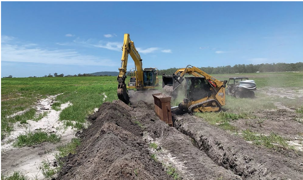
Figure 10. Installing a sub-surface drain.
