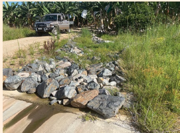
Figure 27. The bottom of a hill with a rock-based water slowing point that connects to the spillway.
