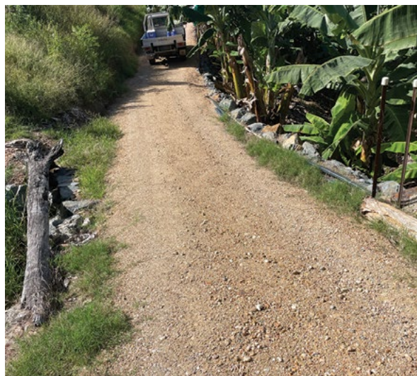
Figure 59. A compacted gravel driveway used to reduce erosion on the main track.
