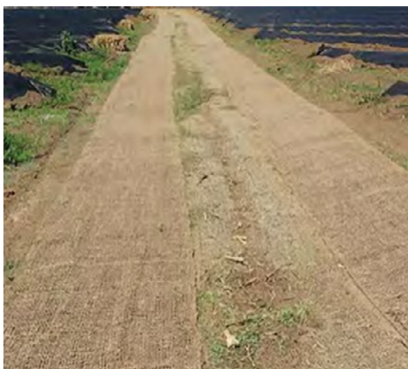
Figure 60. Jute mesh used to line a cross drain. Grass will grow through the mesh and break down afterwards. Photo: C Colmer, Soil Conservation Service.
