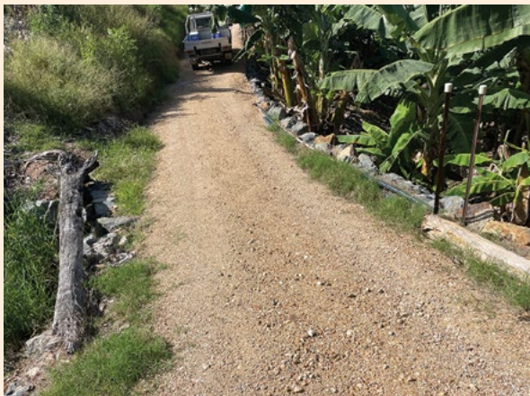
Figure 26. High-quality road gravel compacted and sealed.
