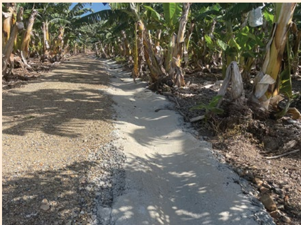
Figure 24. A concrete layer over rocks minimises furrow degradation.
