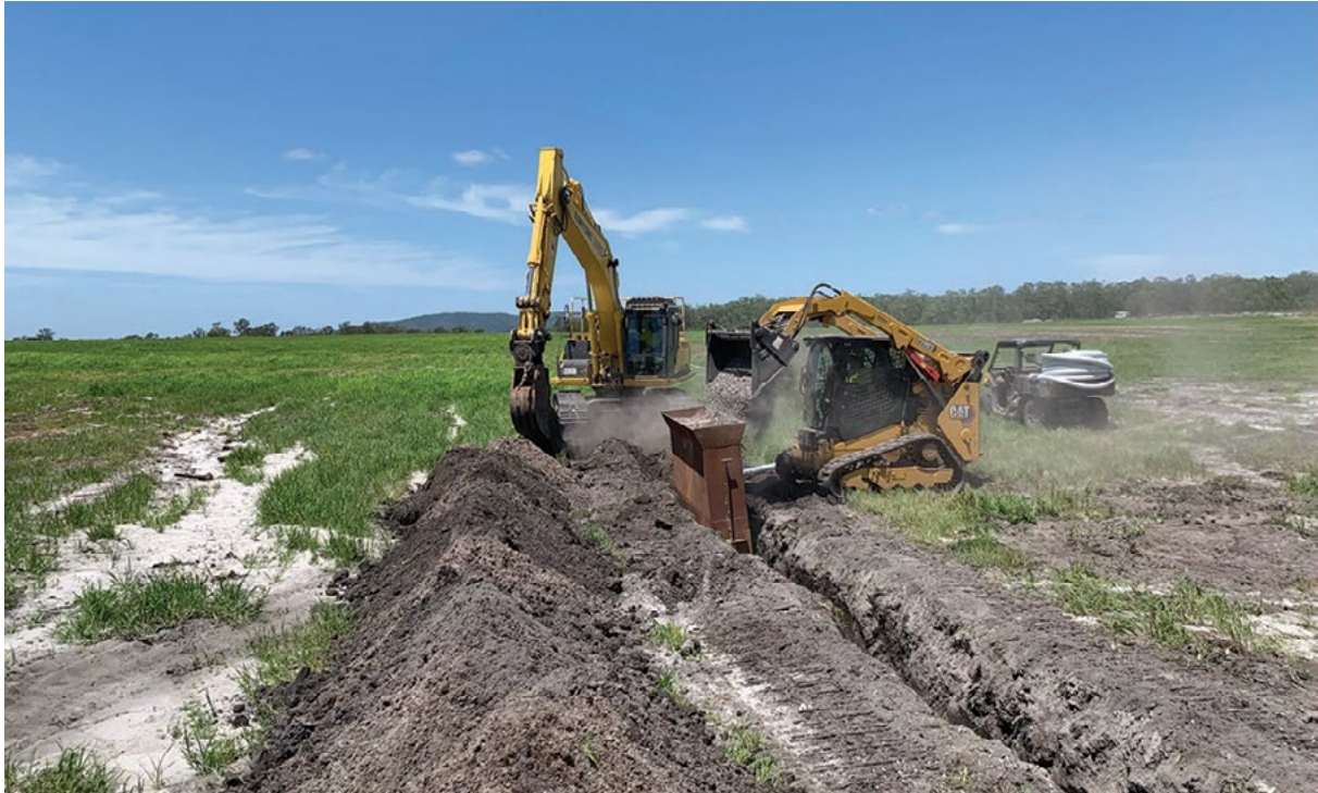
Figure 10. Installing a sub-surface drain.
