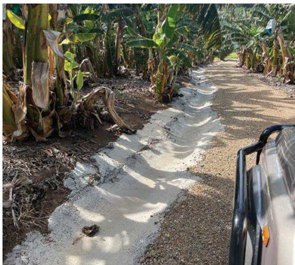
Figure 58. Concrete flume to divert water away from vulnerable slopes.
