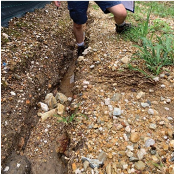
Figure 3. A washout caused by intense rainfall on a blueberry farm.
