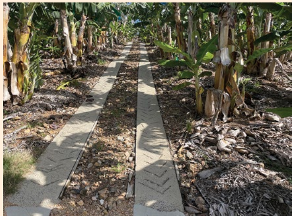
Figure 25. Steep slope concrete tracks with steel reinforcement and pinned to the ground.
