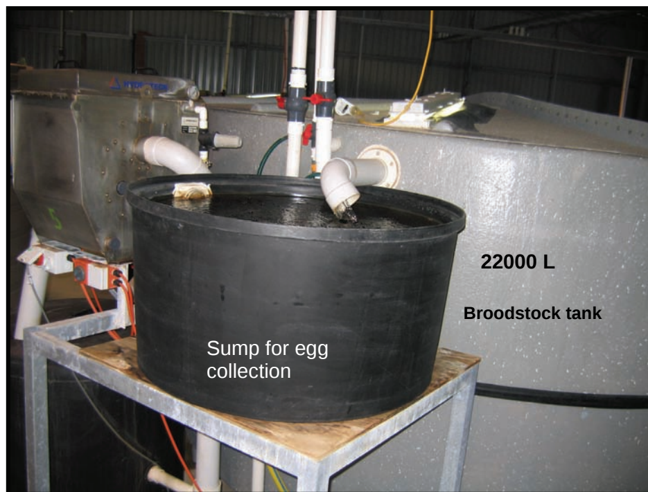
FIGURE 51: Representative broodstock tank used to hold mullet, bass, yellowtail kingfish and snapper at PSFI.
