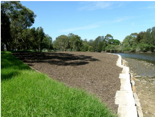
Sandstone blocks replaced deteriorated steel sheet piling to stabilise the banks of the Cooks River. Image Canterbury City Council
